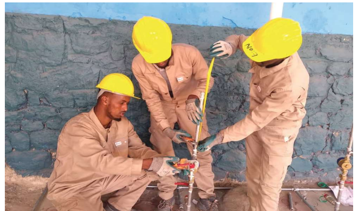
Pharo TVET Plumbing Students
