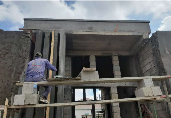
NCD Centre construction in Hargeisa
