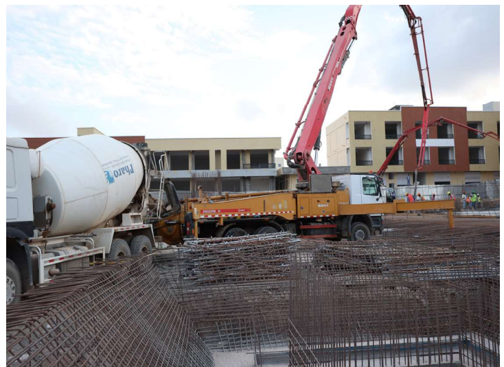
RMC concrete pouring at Waheen Market
